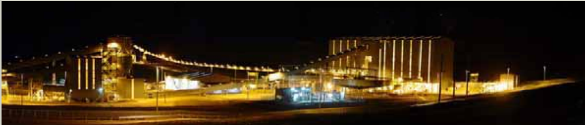
Existing Mt Arthur Coal CHPP
