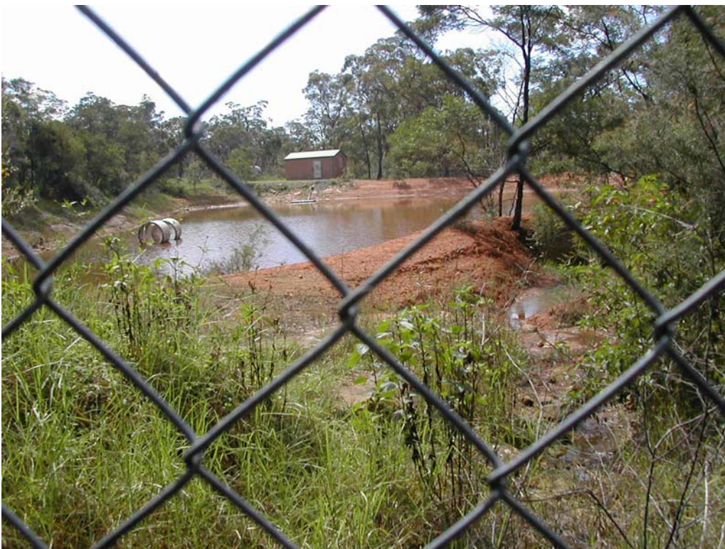
Photo11: Leachate Dam for the former North Nowra Waste Disposal Centre. Looking in a northerly direction on to crown land.
