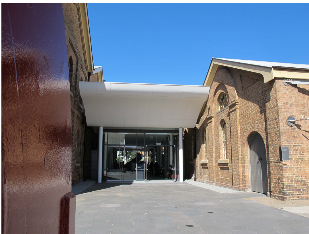
View of existing Newcastle Northern Entrance (Prior to gate installation)
