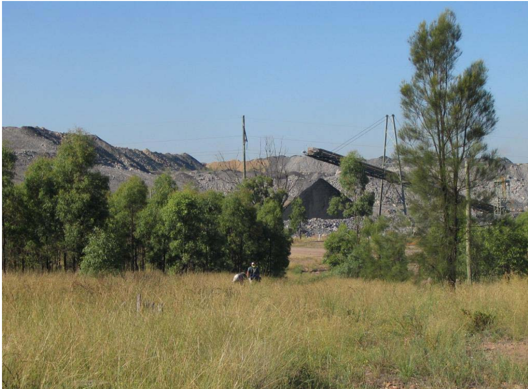
Plate 16 Transects 14, 16 and 17 were undertaken in this general area directly west of the dam. This photograph looking west reveals the heavy disturbance and impact that current mining has caused the general area
