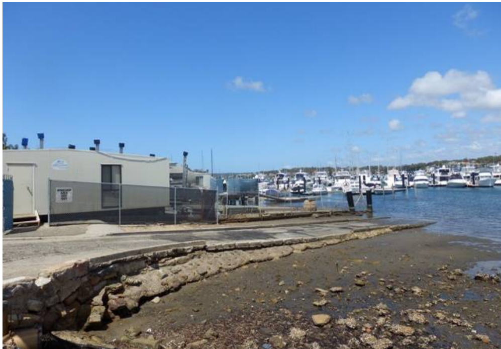
Figure 3-4 View of the northern boundary of slipway area with adjoining Council boat ramp in the foreground
