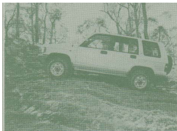
Trafficable cross banks can be comfortably negotiated and provide effective drainage when sited and built correctly.
