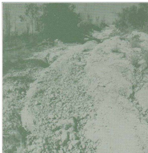
Trafficability is seriously impaired when undrained low standard roads become eroded.
