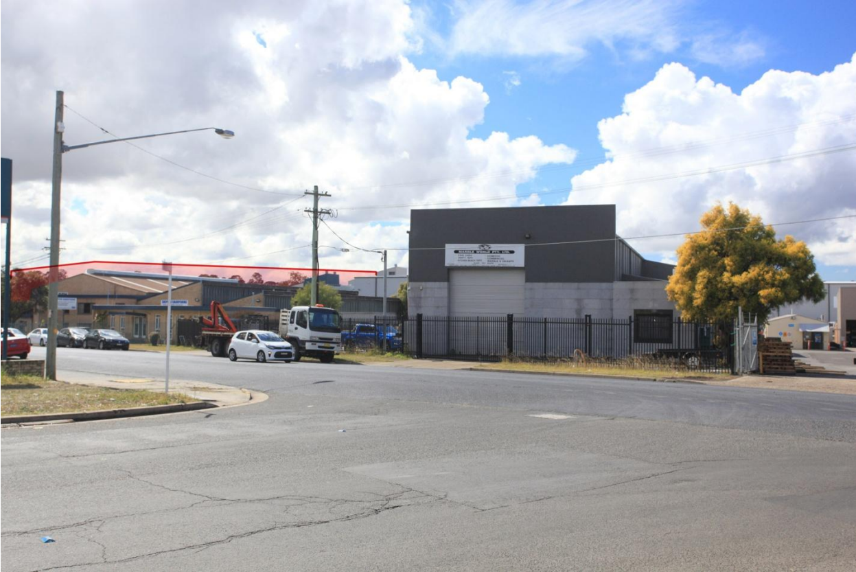
Figure 4.3.1.9 – View Point E
