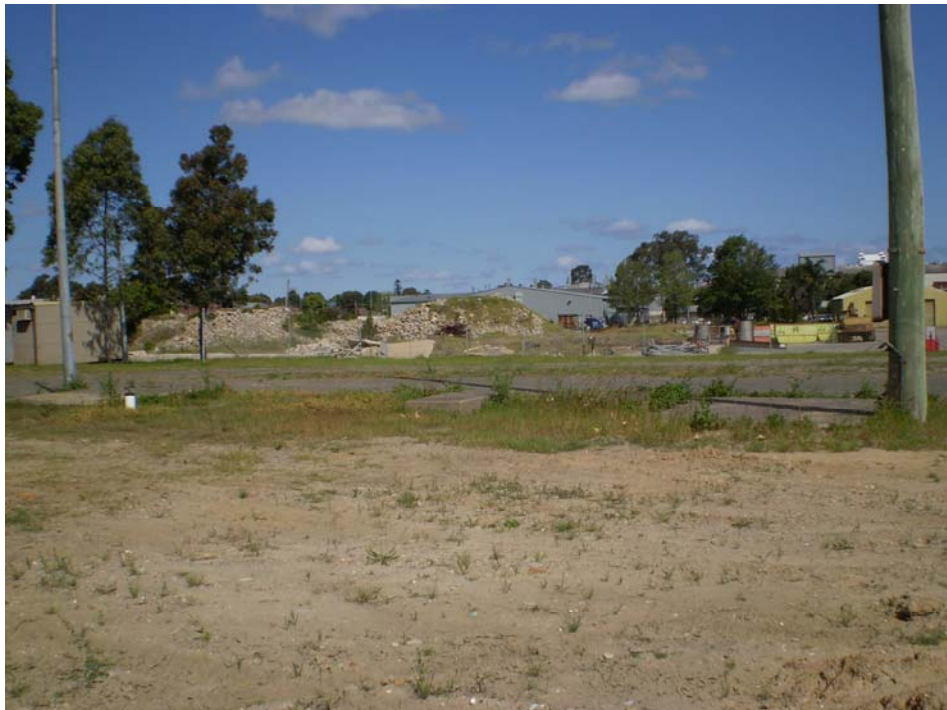
Photo 5- Looking south-east from the location of the removed diesel UST excavation towards the former fuel loading point (sample location TP3).
