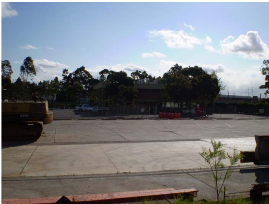
Photo 1- View of two storey office and administration building looking west with office car park immediately to the south and truck parking hardstand area in the foreground.
