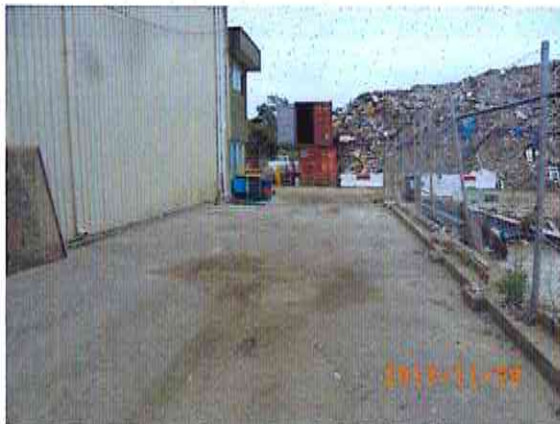
Photo # 177: The current wheel wash area. However, it was observed during the site inspection that a vehicle was being washed in front of the workshop area not in the wheel wash. (refer to Photo # 144).
