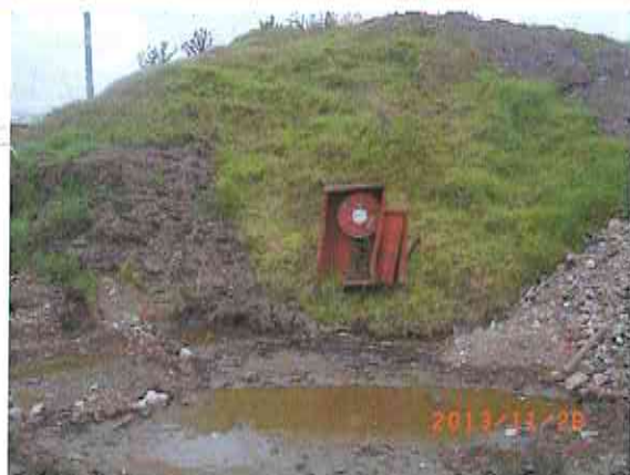
Photo # 240 Stockpile 5: Height of 6.5m, a stockpile with vegetation cover at the most eastern part of the Site.
