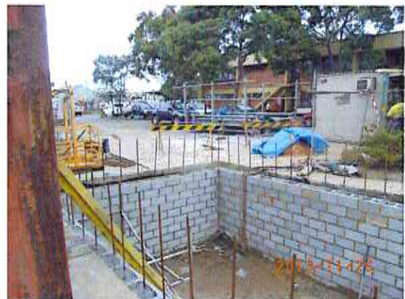
Photo # 366: The new wheel wash and sediment tank area under construction. The wheel wash infrastructure (cattle grid) can be seen the back of the photo.
