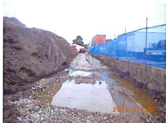
Photo # 241: Internal access road on the eastern boundary of the Site.
