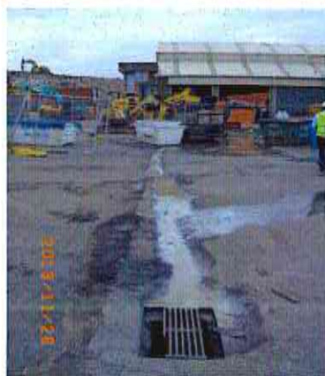
Photo # 144: Runoff from vehicle that was being washed down outside the workshop area into a stormwater drain which drains into the Villawood culvert.
