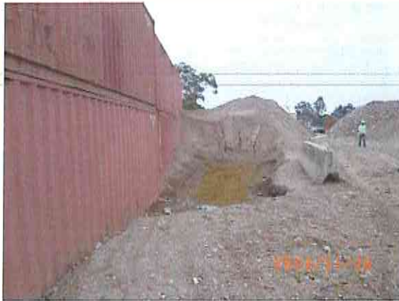
Photo # 232: A sediment dam which had been dug out of waste deposited on site as a stormwater control measure to the west of stockpile 5.
