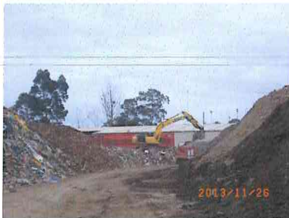
Photo #225: Following sorting of construction waste received on site the residual waste which is not able to be processed into a marketable product is sent off-site to landfill. This photo shows an excavator filling a truck with waste which is being disposed of to landfill.
