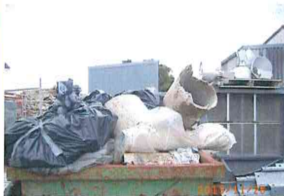
Photo # 154: Waste material (fibro cement potential ACM) stored in skip bins on the south western corner of the Site.
