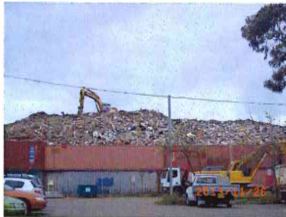
Photo # 118: Stockpile 1: Height of 11.5m, located in the centre of the Site, refer to aerial in Section 4.1, consisting of unprocessed waste.
