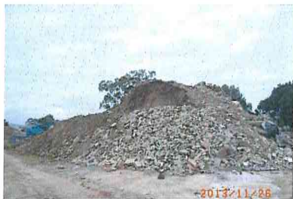
Photo # 213: Stockpile 2: Construction materials sorted into bricks and concrete.
