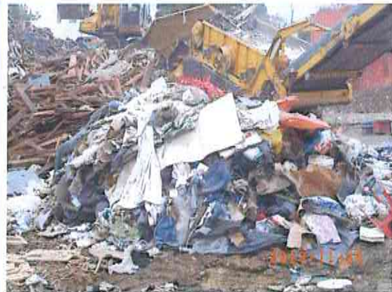
Photo # 329: Close-up shot of residual waste sent to offsite landfill.
