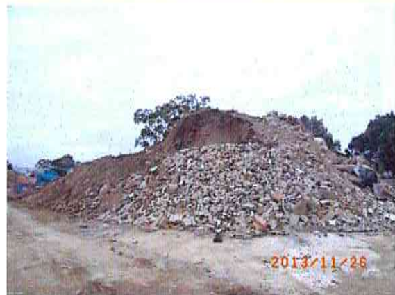
Photo # 217: Stockpile 2: Height of 8.0m, located in the southern corner of the Site, refer to aerial in Section 4.1. Made of separated brick, concrete and gravel materials, ready for processing.
