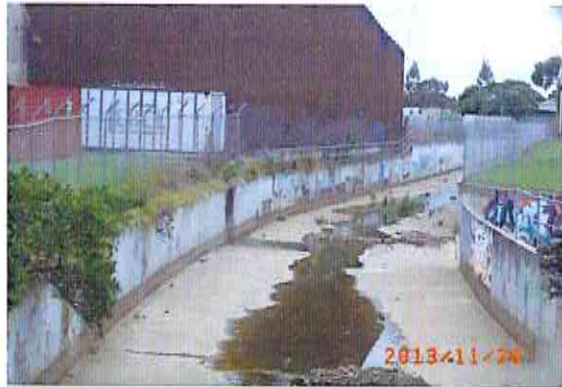
Photo # 104: Villawood culvert (offsite). Site discharge pipe on left wall.
