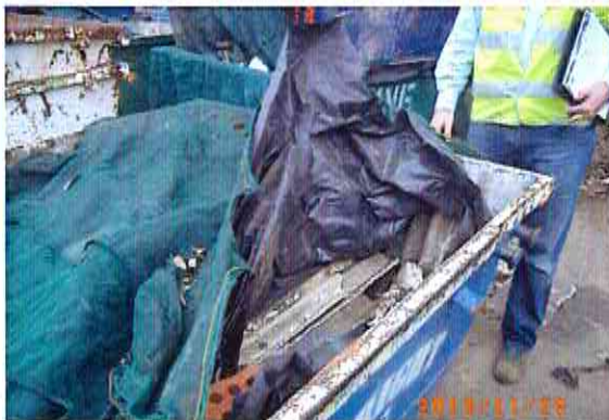
Photo # 200: Waste material (potential ACM) stored in skip bins on the south western corner of the Site.
