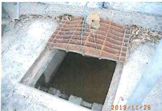
Photo # 098: The final drainage point on site to the Villawood culvert.
