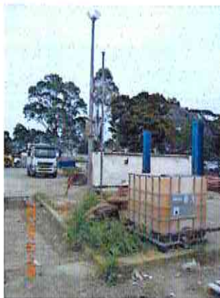
Photo # 206: A vent pipe and fill/dip point metal gatic cover was observed along with a raised concrete pad at the western end of the Site. No bowser dispenser was observed on or near the raised concrete pad, which suggests that refuelling activities are no longer undertaken. However the presence of the surface infrastructure may indicate the presence of underground storage tanks, which may contain fuel.
