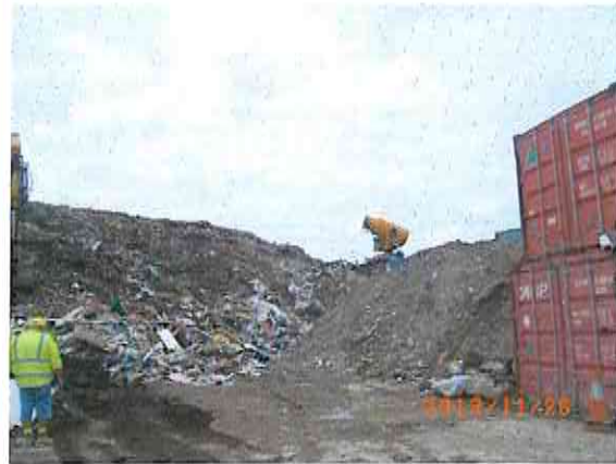
Photo # 353: Fogging machine is used for dust suppression over stockpile 1, and where waste is received and processed.
