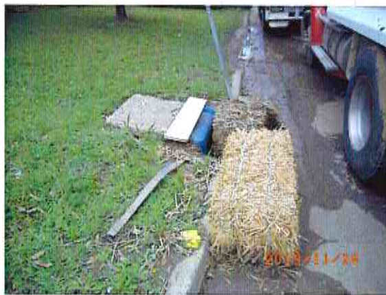
Photo # 110: Stormwater drain on the driveway, near the visitor's car park. Covered with hay bales as a sediment control measure.
