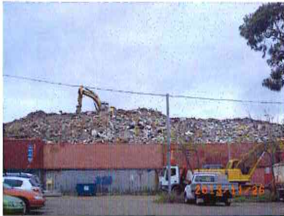
Photo # 118: Shipping containers on the perimeter of the waste processing area.
