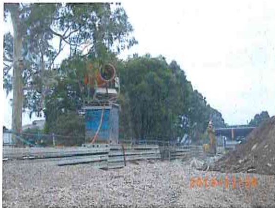
Photo # 261: One of two fogging machines used on site to reduce dust emissions from the Site. Also note in this picture the temporary noise bund, which will reportedly be constructed into a noise bund at the southern boundary of the Site.
