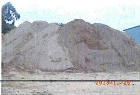
Photo # 220: Stockpile 3: Height of 5m, containing soil on the southern boundary of the Site. Sorted and processed.
