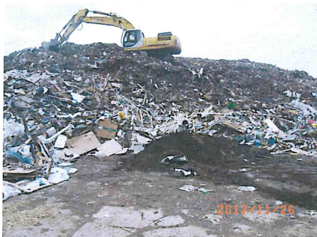
Figure 5 – Machinery operating on top of a stockpile
