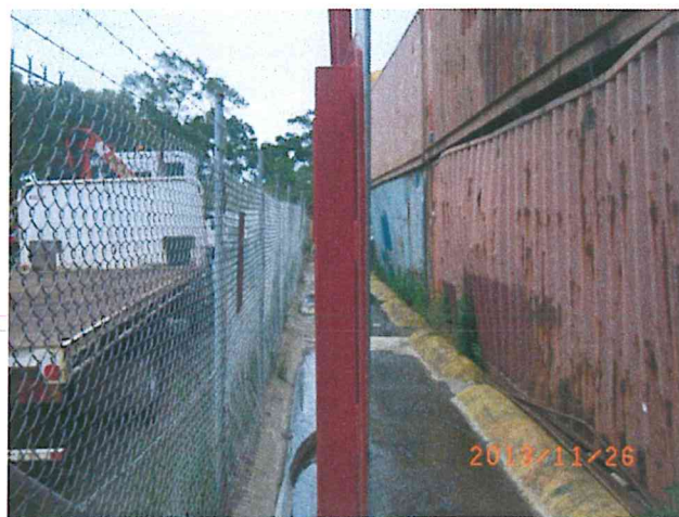
Figure 8 – Rusting container stacks
