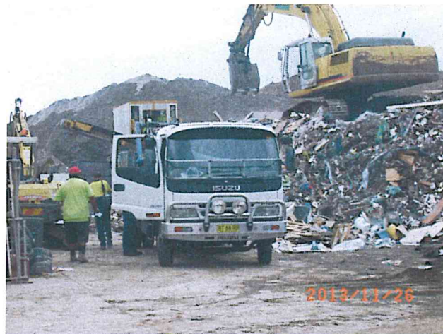
Figure 6 – Machinery operating on top of a stockpile
