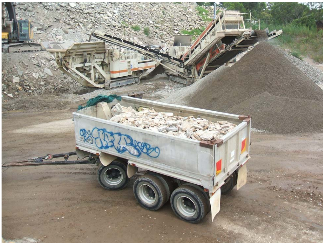
Figure 6 Concrete Crushing Operations and Aggregate Storage at a Materials Processing Facility
