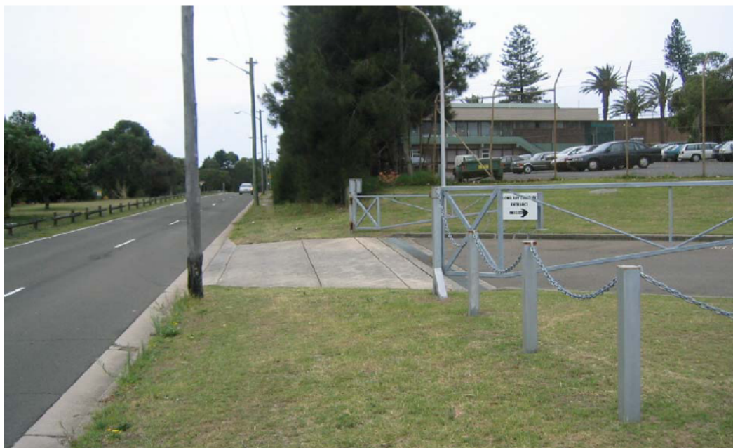
View of the existing entry driveway from Anzac Parade.
