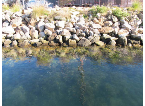
Rock revetment behind the existing north-south floating pontoon
