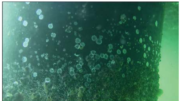
The top of piles located underneath the floating pontoons lacked the macroalgae and oysters present under the wharves and were dominated by small barnacles and microalgae.
