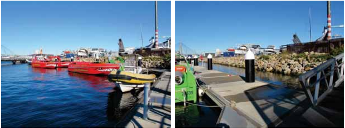
Existing north-south marina pontoon to which the proposed finger wharf will be attached.
