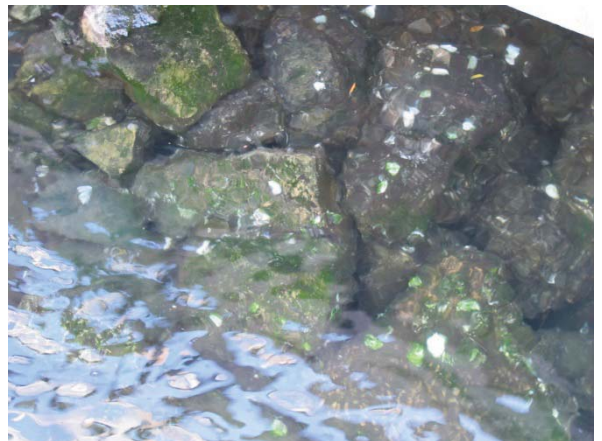
Rock revetment behind the existing north-south floating pontoon
