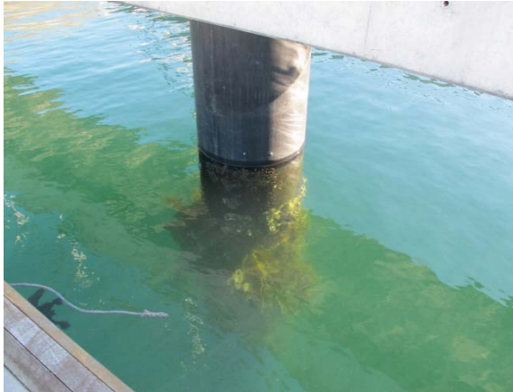
The top of HDPE piles located underneath the wharves with rock oysters and Ecklonia sp.
