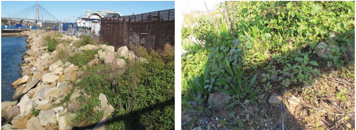
Exotic plant species were found growing along the riparian zone of the rock revetment.
