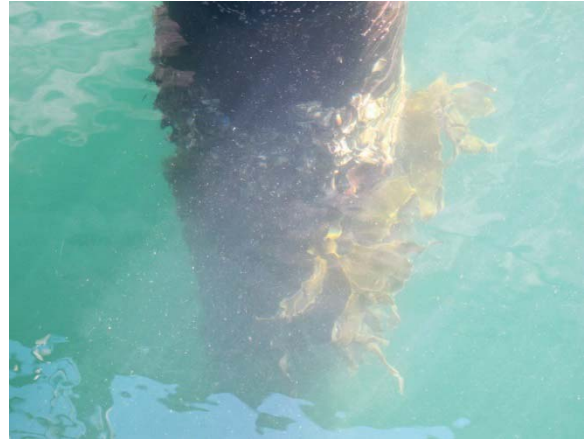
The top of HDPE piles located underneath the wharves with rock oysters and Ecklonia sp.
