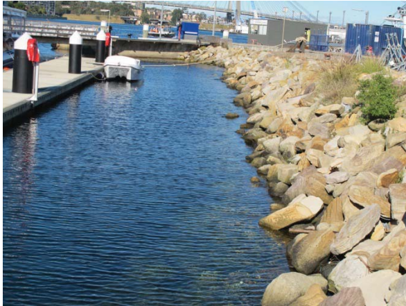
Rock revetment behind the existing north-south floating pontoon
