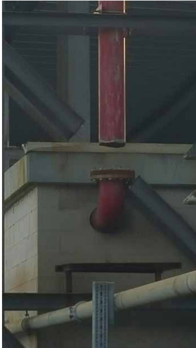
PHOTO 7: Existing Steel Gantry bracing cut in location of proposed Cantilevered Roof
