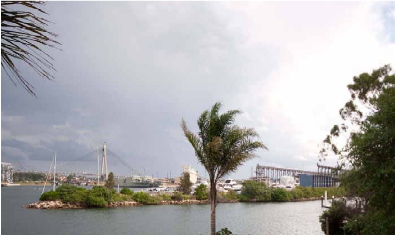
Figure 5.5 PO1 from public walkway at Balmain East – current approved and built
