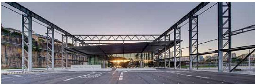
IMAGE 3: Existing steel gantry used integrally at White Bay Cruise Terminal - image by others
