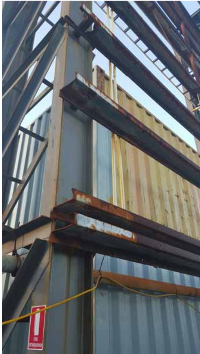
PHOTO 6: Existing Steel Gantry girts in location of proposed Cantilevered Roof
