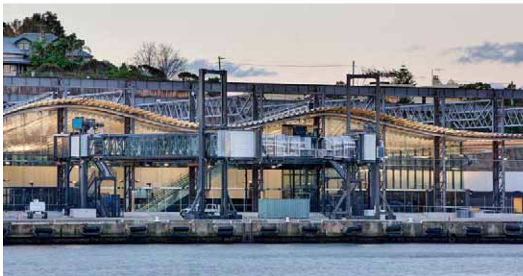
IMAGE 2: Existing steel gantry used integrally at White Bay Cruise Terminal - image by others
