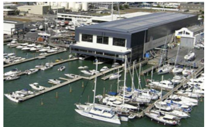
Fig. 17 - internal shed and external holding area
