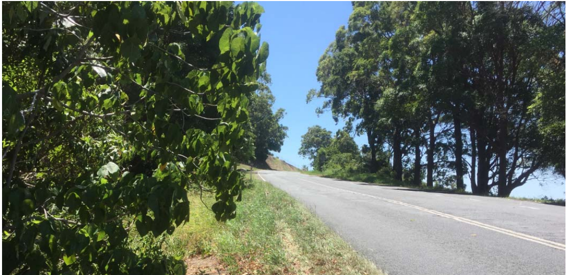
Figure 4: Example of existing trees within the clear zone
