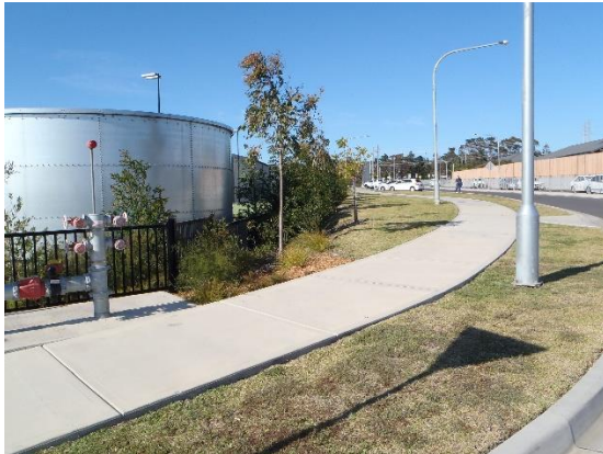
Photo 1: View of existing sprinkler water tank and landscaping at boundary of site to roundabout in Moona Creek Road – refer to Zone D existing features in architectural drawings at Appendix A. The proposed timber screen shown in Zone B in the architectural drawings at Appendix A, will be located on the outer face of the existing palisade fence within the site boundary. Existing landscaping to remain.
