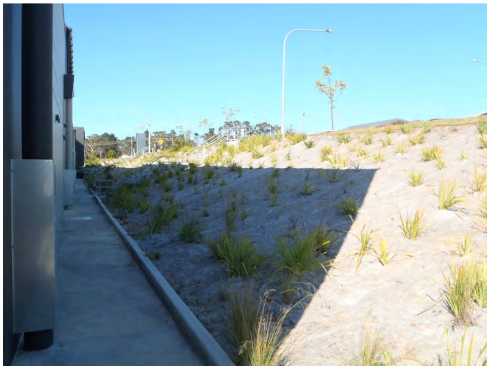
Figure 8. The Moona Creek Road embankment (above and below – both photos looking southwest), proposed for additional tree, shrub and plants along with topsoil and bank stabilisation coir logs as proposed on plan L_101
