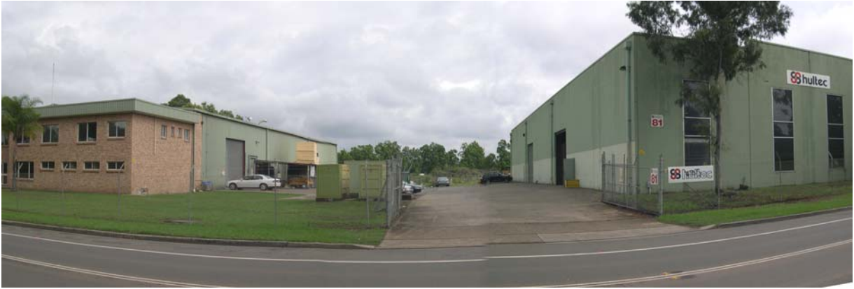
View of the site from Christie Street
