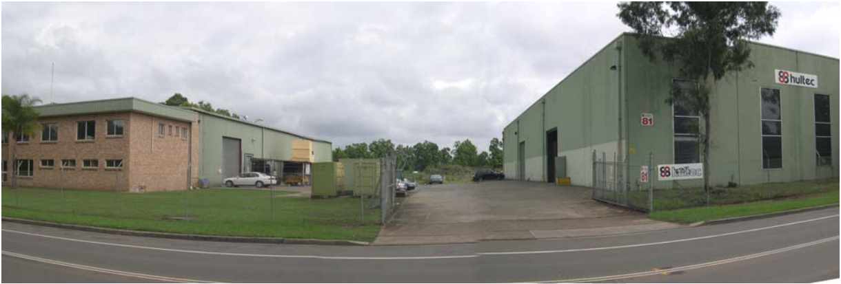
View of the site from Christie Street
