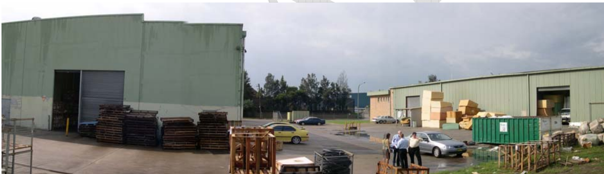
View towards Street from the proposed location of the facility
