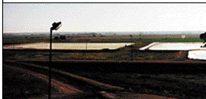
Photo 1. Three of the eight lined containment ponds: An evaporation pond is pictured on the left side of the photo, while two intermediate quality ponds are visible on the right.
