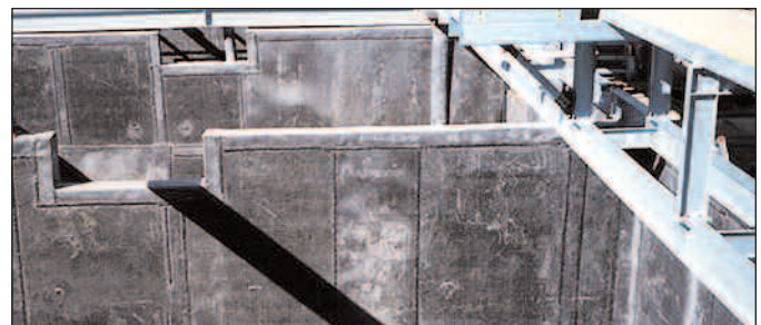
HDPE liner deployed over concrete in a wastewater treatment aerobic digester.
