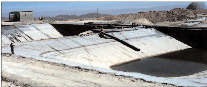
White Surface HDPE Geomembrane liners utilized for Industrial waste processing ponds.
