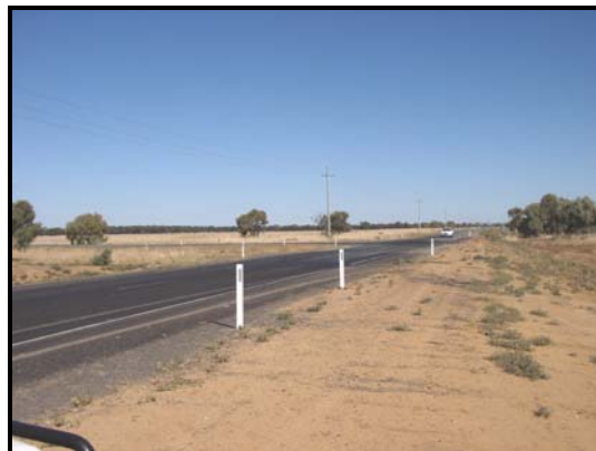
Plate 11: Kidman Way / Eulo Road Intersection (northern approach)
