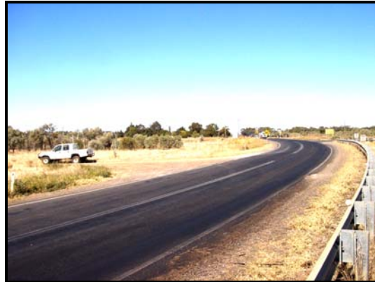
Plate 26: Willbriggie Railway Crossing (northern approach)
