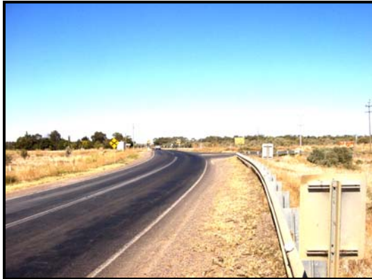
Plate 25: Willbriggie Railway Crossing (northern approach)
