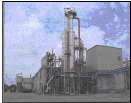
Plate 2: Indicative Ethanol Plant Construction
