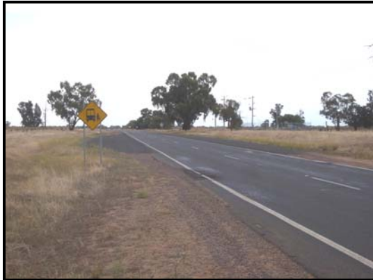
Plate 8: Kidman Way / Ringwood Road Bus Stop (southern approach)
