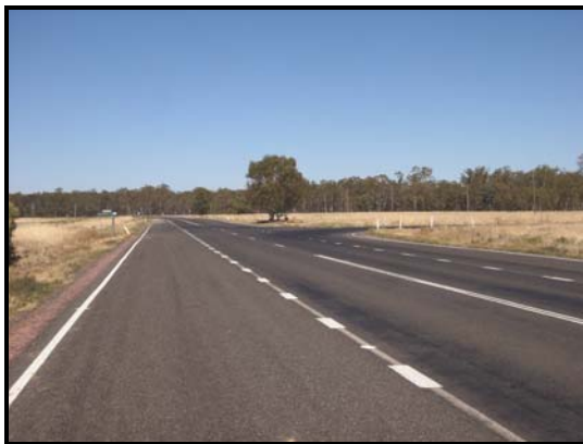
Plate 27: Kidman Way/River Road Intersection (northern approach)
