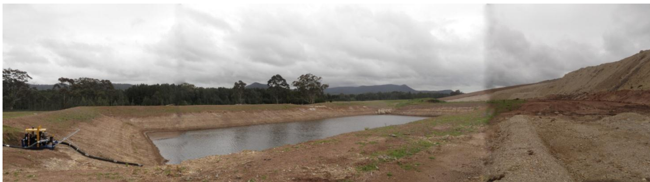
Figure 2.7 Northern Out of Pit (NOOP) Sediment Dam
