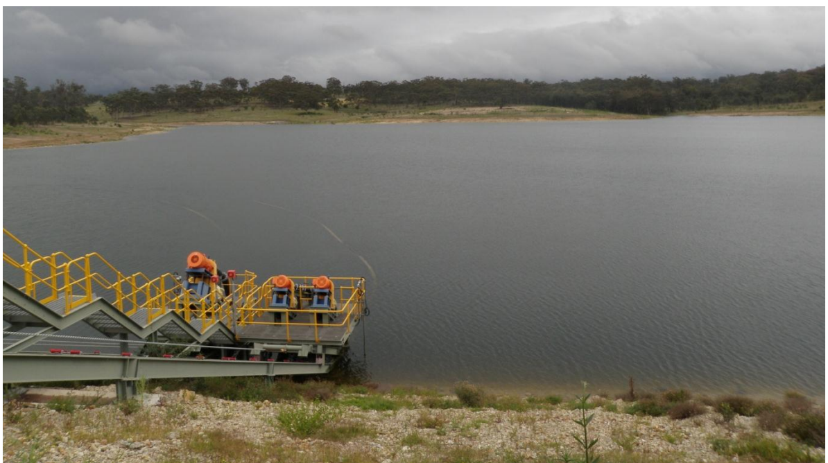
Figure 2.6 Raw Water Dam
