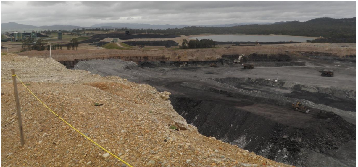
Figure 2.5 Pit Water Dam (in background)
