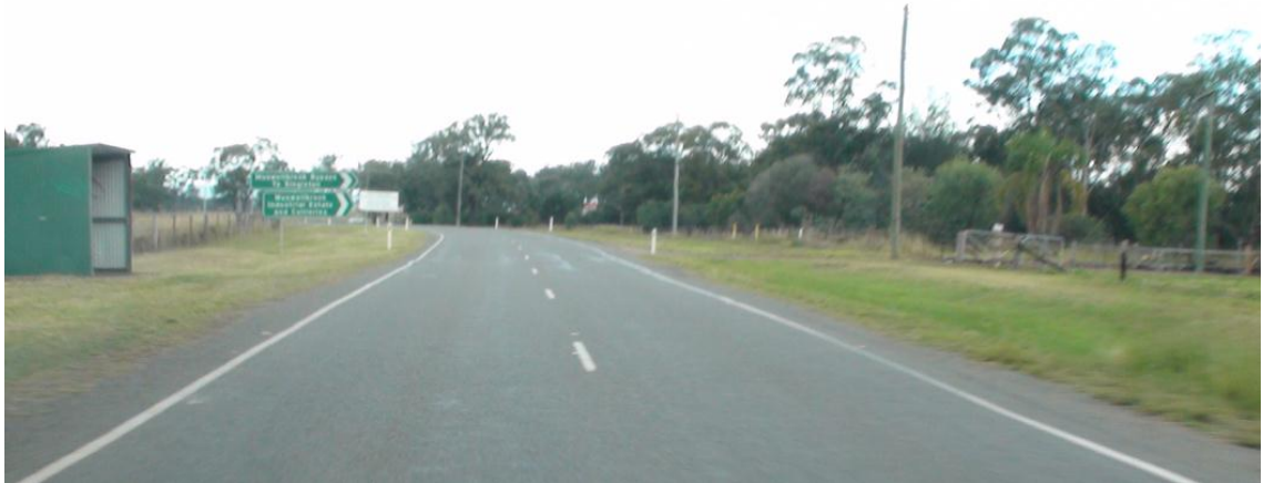
Figure 2-4 Denman Road, looking east towards Thomas Mitchell Drive
