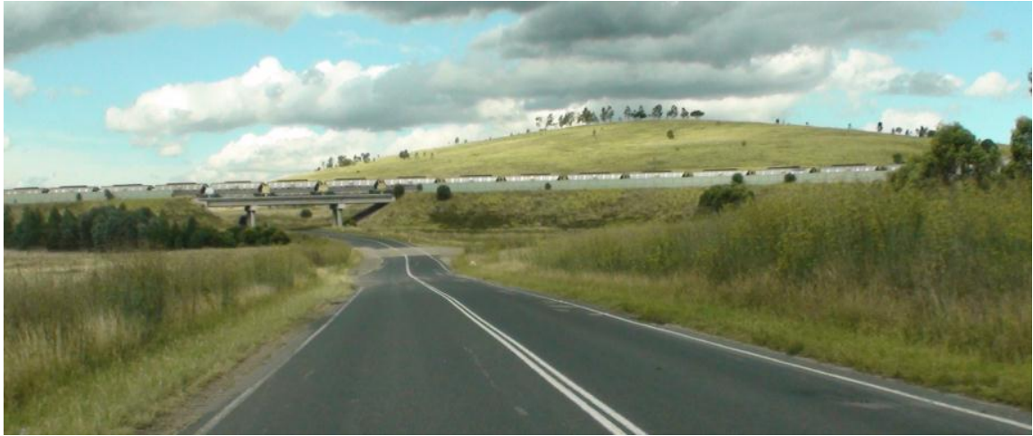
Figure 2-5 Thomas Mitchell Drive, looking south towards railway overbridge at MAC
