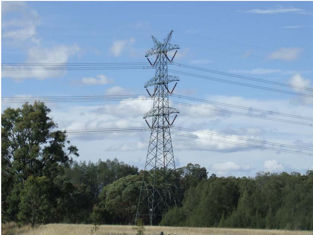
P2 – Viewing distance to tower 200m
