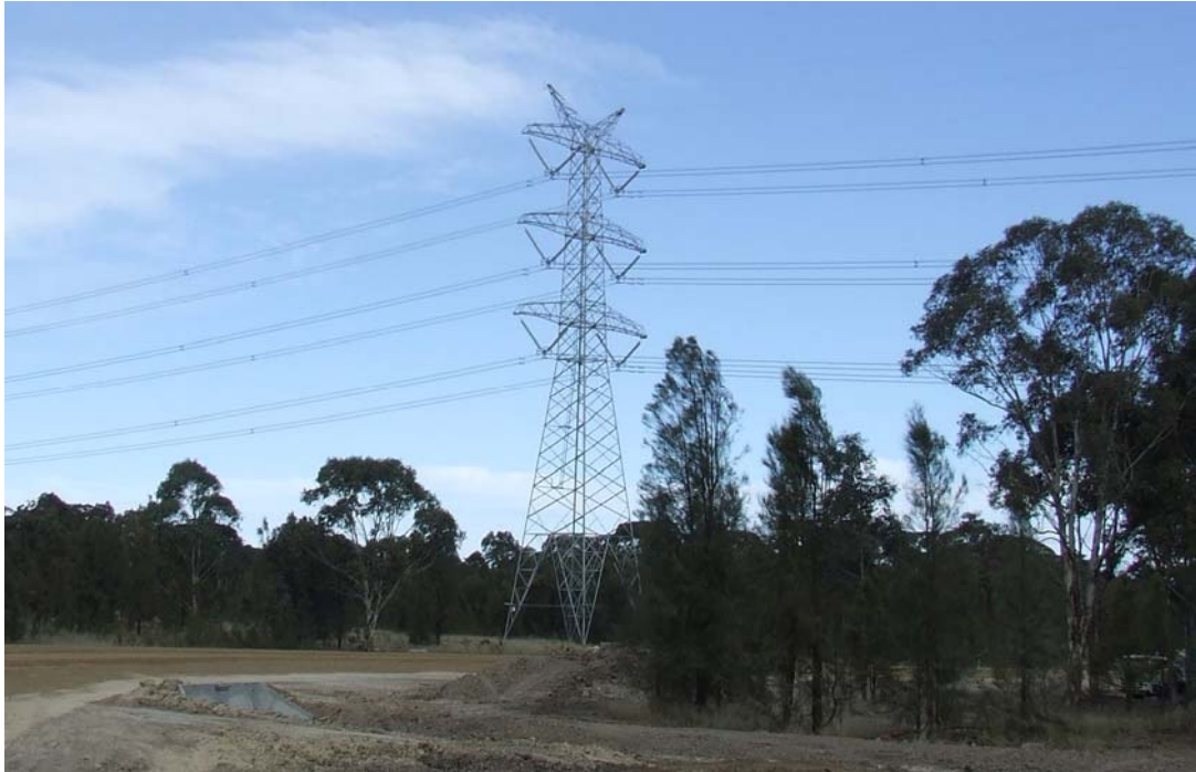
P9 – Disturbed area
