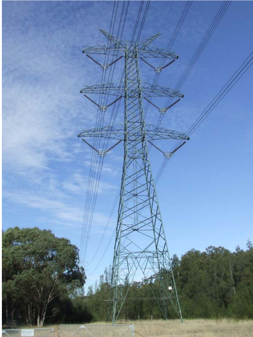
P1- Distance to tower less than 100m immediately adjacent to the road
