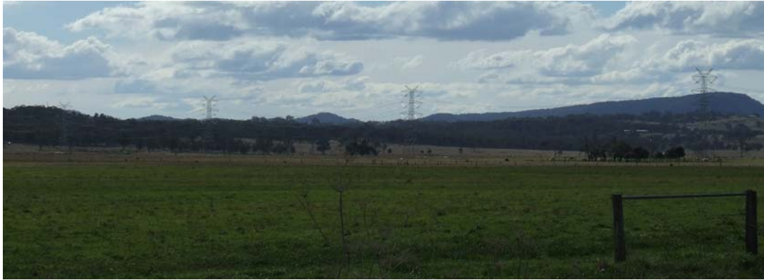
P6 – towers partially visible against background
