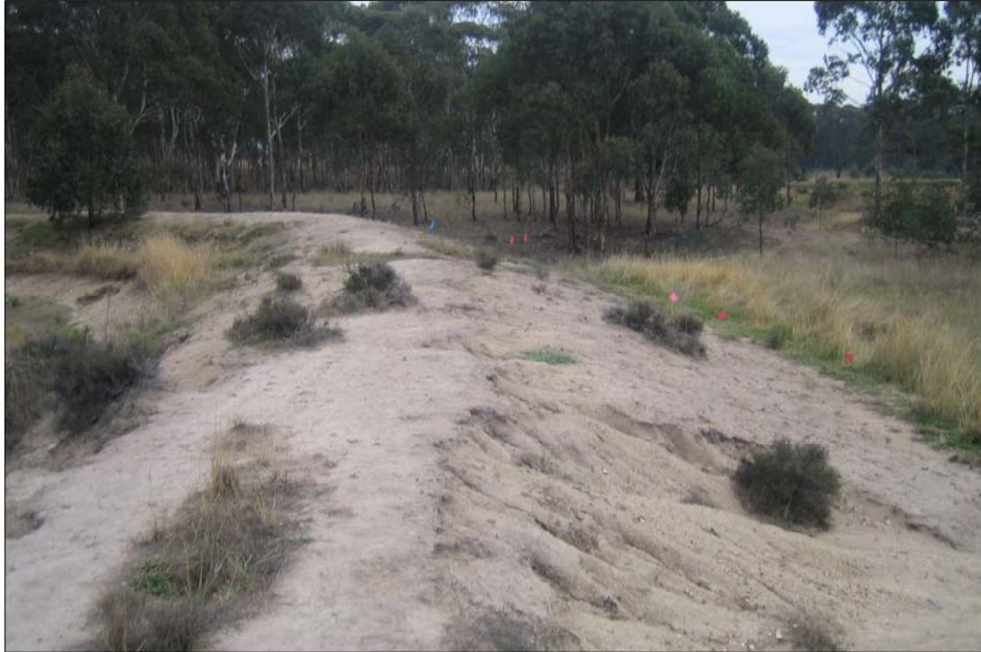
PLATE 5 BFC75 site on bank of dam
