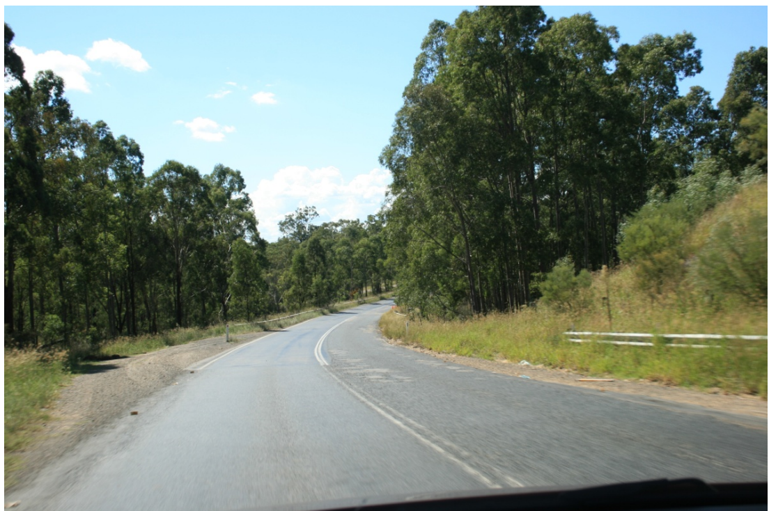
Figure 2.32 Substandard curve with no sufficient delineation provided - Thomas Mitchell Drive, looking eastbound
