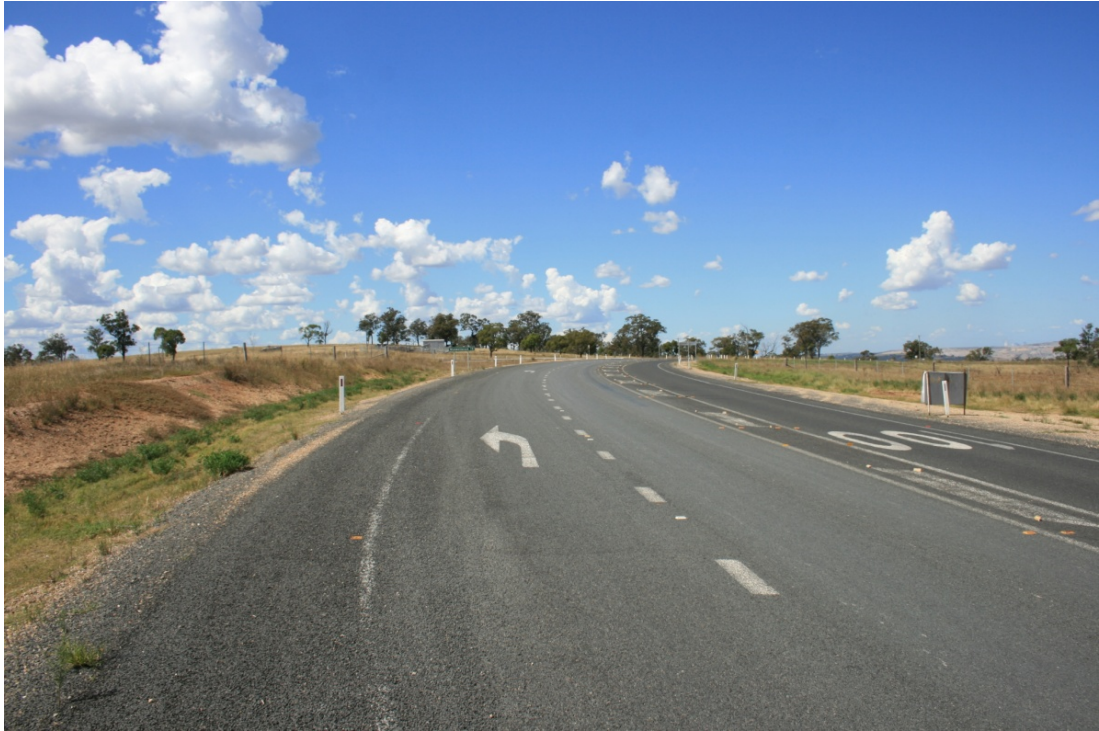
Figure 2.22 Edge line covered with chipseal aggregate - Wybong Road, looking eastbound toward its intersection with Bengalla Link Road
