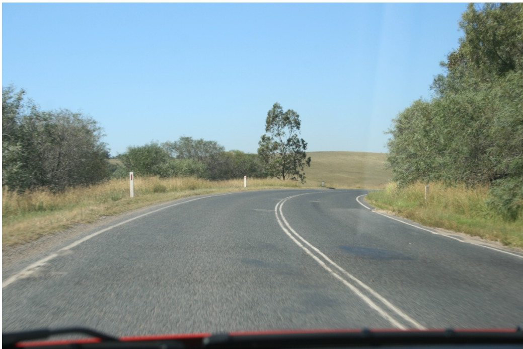
Figure 2.30 Substandard curve with no sufficient delineation provided - Thomas Mitchell Drive, looking eastbound
