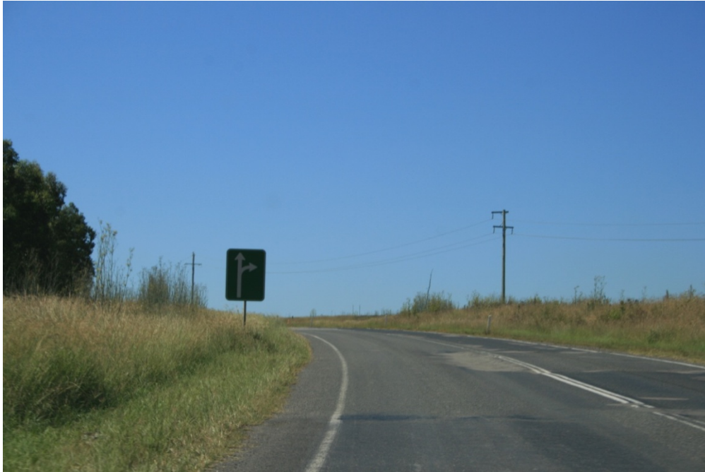
Figure 2.33 Substandard curve with no sufficient delineation provided - Thomas Mitchell Drive, looking eastbound
