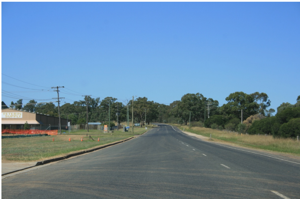
Figure 2.28 No edge line painted - Thomas Mitchell Drive, looking eastbound
