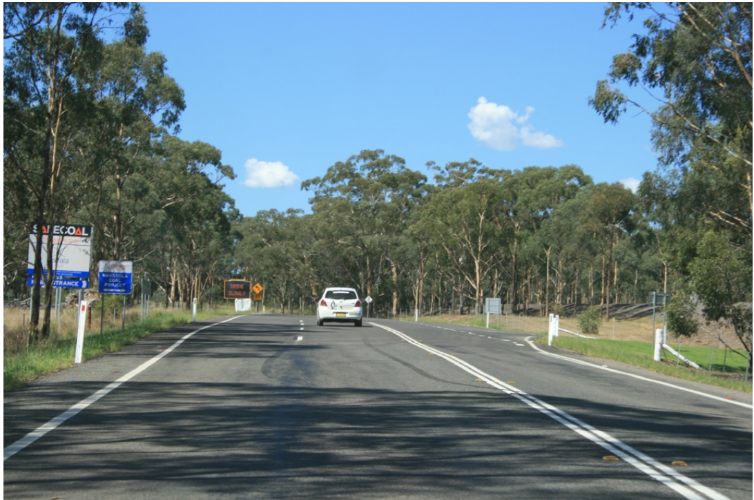
Figure 2.14 Bengalla Link Road/Wybong Road intersection
