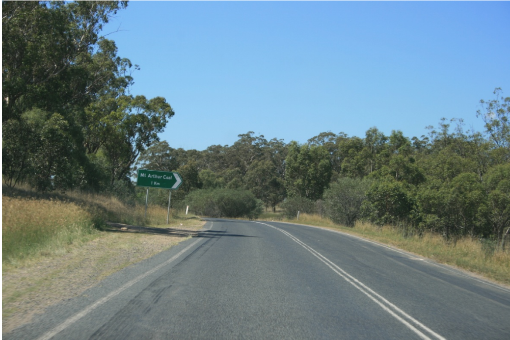
Figure 2.29 Substandard curve with no sufficient delineation provided - Thomas Mitchell Drive, looking eastbound
