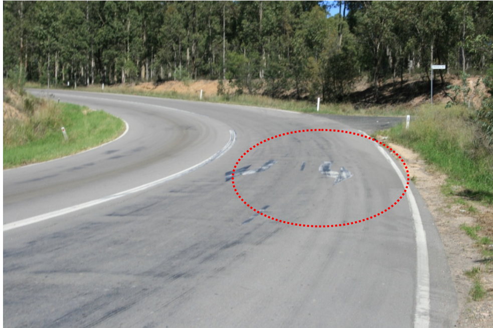
Figure 2.34 Pavement arrows covered by tyre marks - Thomas Mitchell Drive, looking westbound, on approach to its intersection with the New England Highway
