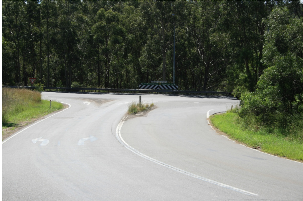
Figure 2.9 Thomas Mitchell Drive, on approach to its intersection with New England Highway
