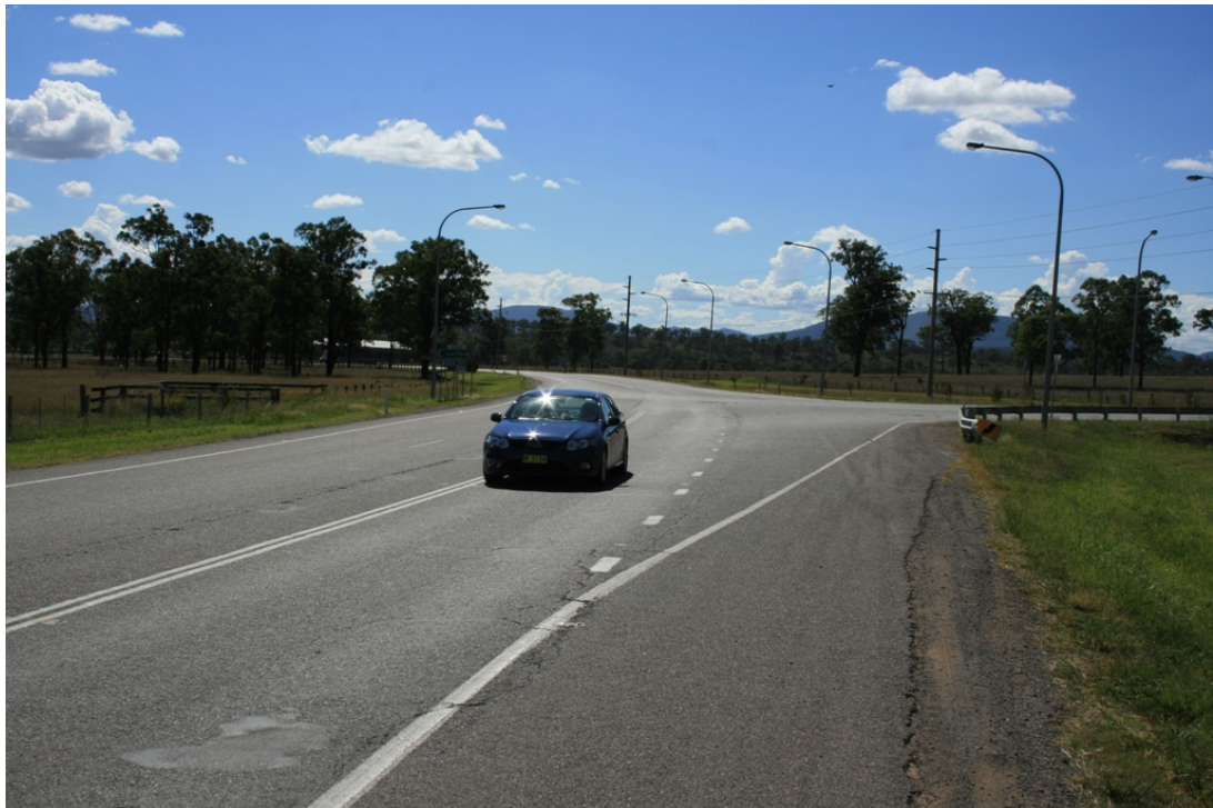
Figure 2.10 Denman Road/Thomas Mitchell Drive intersection
