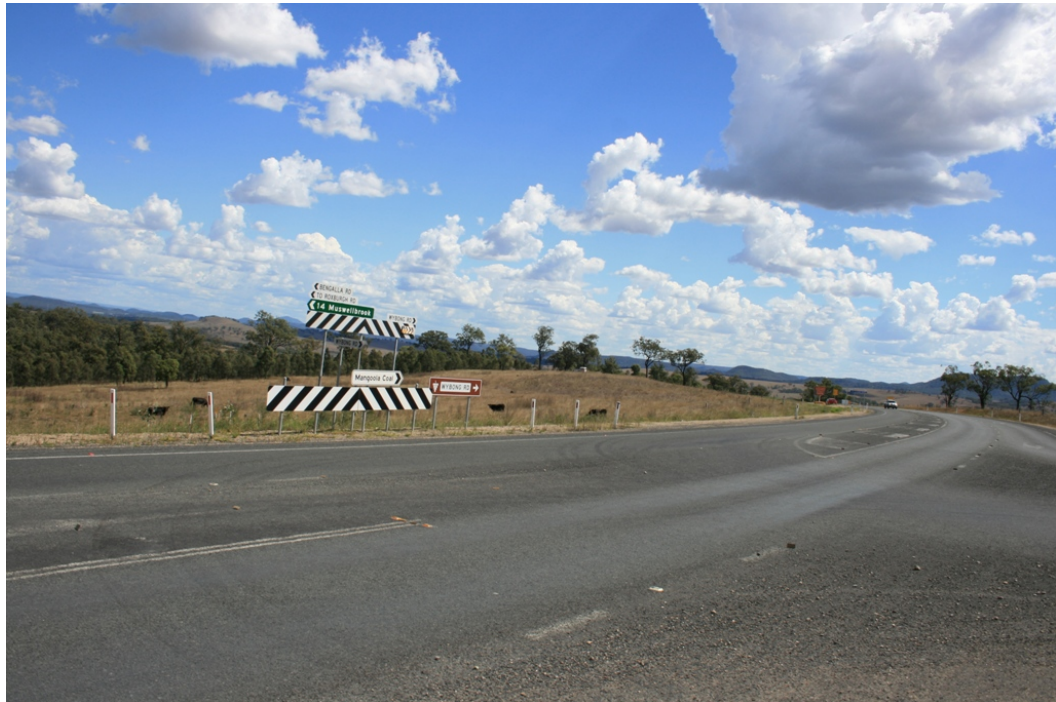
Figure 2.13 Bengalla Link Road/Wybong Road intersection
