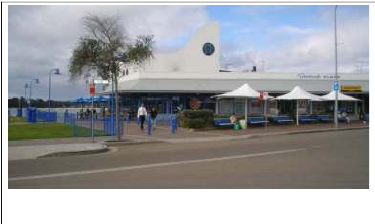
Figure 9: Foreshore development to south east, Clyde Street
