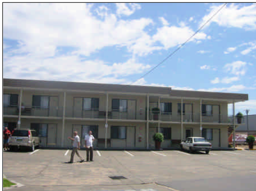
Figure 7: View of the western-most wing of the existing motel, looking west from within the site
