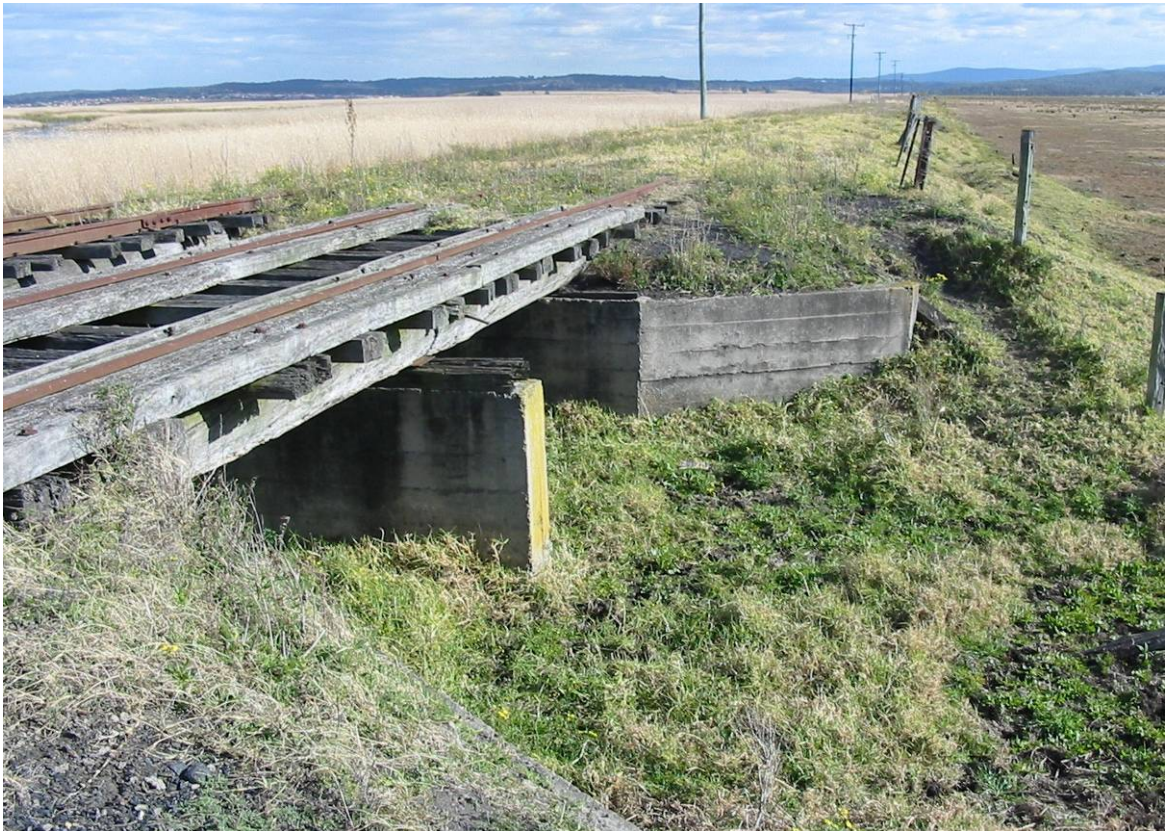
Figure 2.7 Typical culverts under Richmond-Pelaw Rail line
