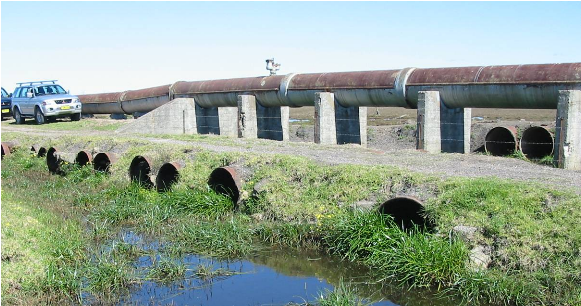
Figure 2.13 Typical access along Hunter Water pipeline with culverts that may need to be replaced (subject to individual assessments during works activities)
