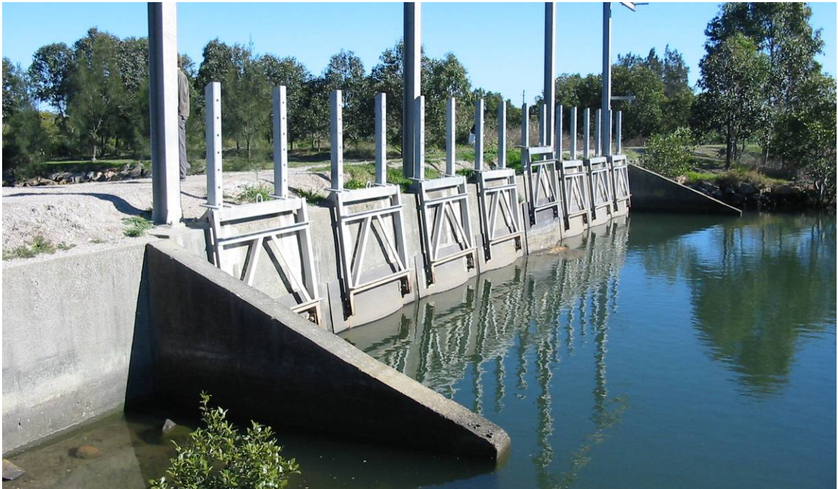
Figure 2.1 Existing Ironbark Creek Floodgates
