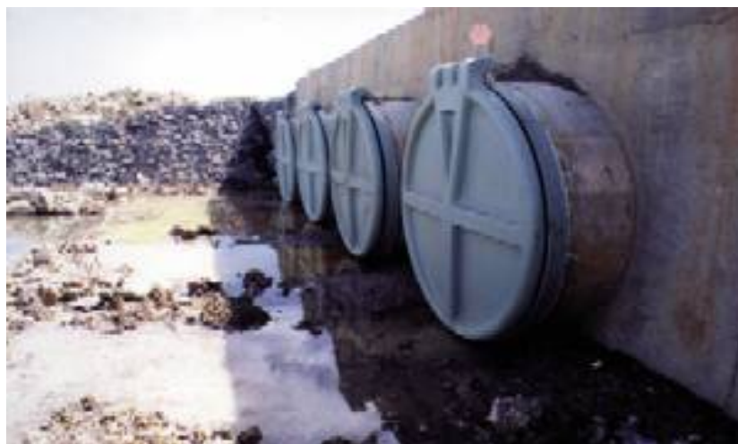
Figure 2.19 Example of typical flapgates proposed for Hexham Swamp drains (source: www.humes.com.au )
