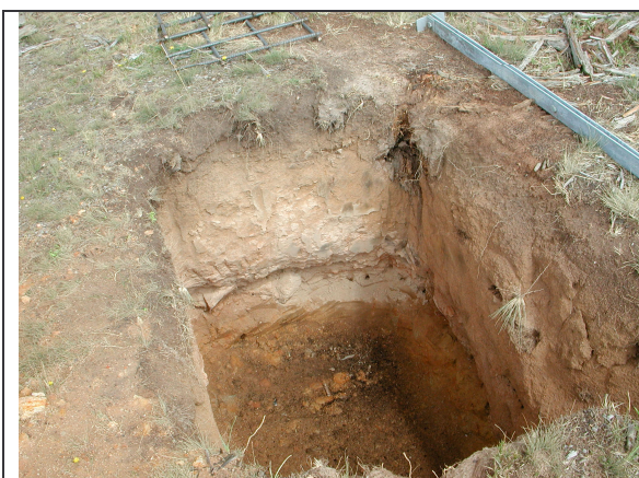
Plate 5.8 – Footing for Hammonds Hill Monitoring Tower
