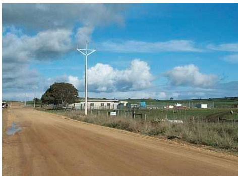
Plate 3.2 Typical Site Office and Storage Area
