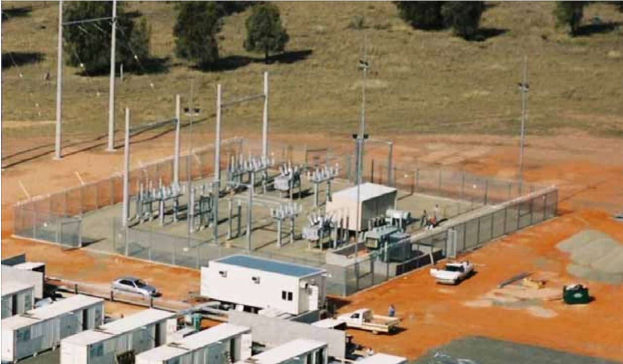
Figure 3.9 Typical single-transformer substation
