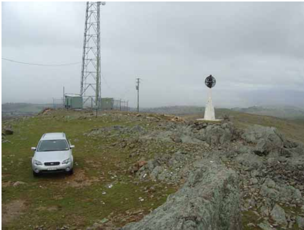
Figure 7.7 Black Trig Communications tower
