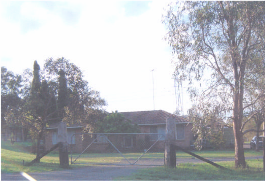
Photo 2 Transgrid lines behind house (Note Integrals line are to the left – see Photo1)
