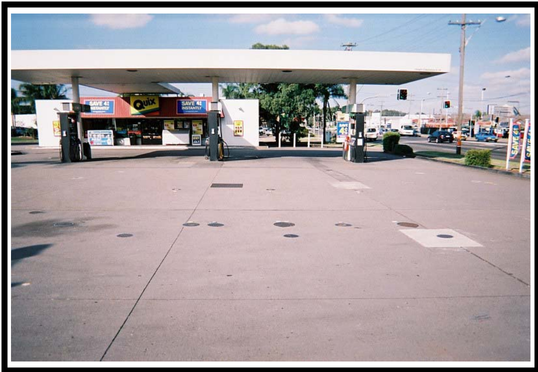
Photo 4: Looking east towards sales building and canopy. Tankfarm in the foreground.
