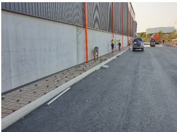
Photo 17. 18/12/2019 – Looking south-west along bitumen surfaced access road on western extent of site.
