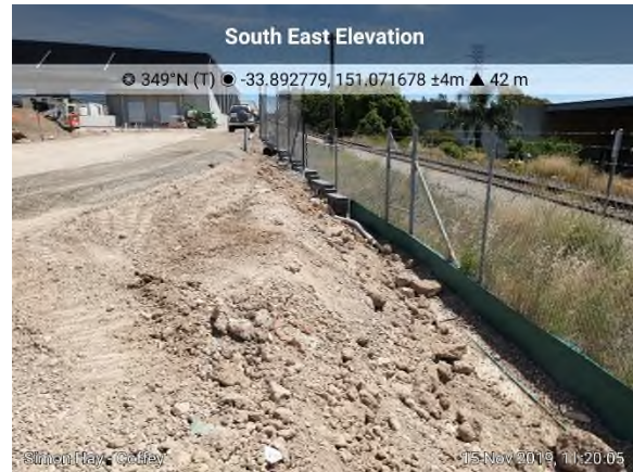
Photo 2. 15/11/2019 – Looking north-west along eastern boundary of Precinct H, depicting VENM cap thickness (approximately 1m) and railway corridor further east.
