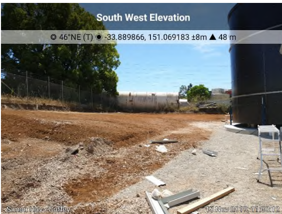
Photo 9. 15/11/2019 – Looking north-east at cap clay capped surface at rear of fire pump room and water tank.
