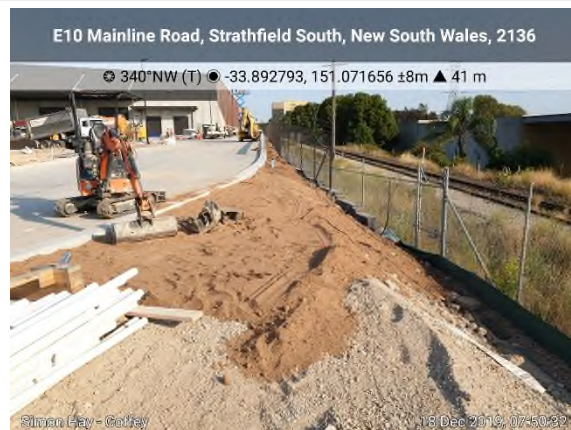
Photo 16. 18/12/2019 – Looking north-west across capped surface of H1 at imported topsoil.
