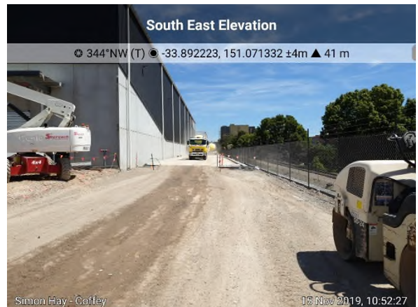
Photo 4. 15/11/2019 – Looking north-west along eastern boundary of Precinct H, at paved internal access road.
