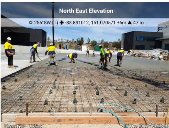
Photo 5. 15/11/2019 – Looking south-west across central loading dock area located between H1B and H2 warehouse as concrete slab over VENM cap was being poured.
