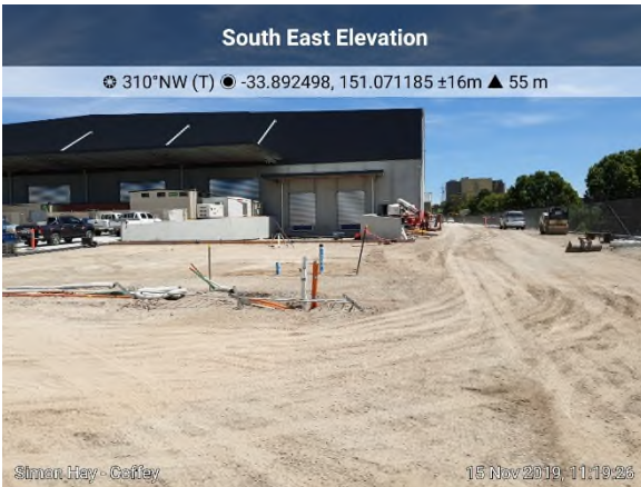
Photo 1. 15/11/2019 – Looking north-west across Precinct H at H1A warehouse, with VENM capped surface in foreground.
