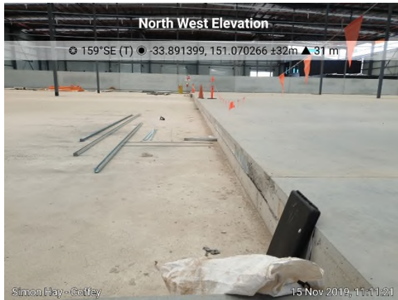
Photo 13. 15/11/2019 – Looking south-east across capped surface of H1B showing an approximate concrete cap thickness of 300mm on right side of photograph.
