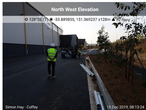
Photo 24. 18/12/2019 – Looking south-east along western border of site at bitumen surfaced internal road and landscaped areas along western border adjacent to rail corridor.
