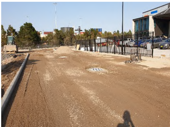
Photo 15. 18/12/2019 – Looking west across southern portion of H1 carpark prior to surfacing.
