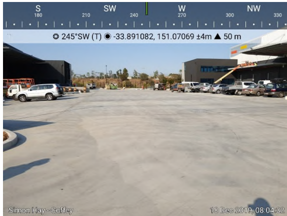
Photo 19. 18/12/2019 – Looking west / south-west at loading dock forecourt between H2 and H3 warehouses.
