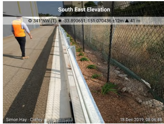
Photo 20. 18/12/2019 – Looking north-west along eastern border of site with mulched landscaped border and hardstand (7mm Prime and Seal) internal road.
