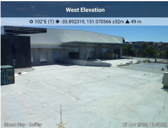
Photo 7. 15/11/2019 – Looking east at warehouse H2 at concrete surfaced loading dock area.
