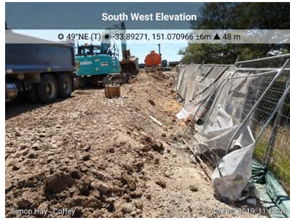
Photo 14. 15/11/2019 – Looking north-east across capped surface of at southern end of Precinct H showing approximately VENM cap thickness of 1m.
