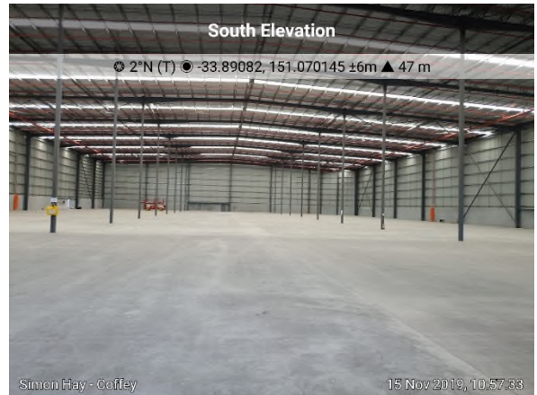
Photo 8. 15/11/2019 – Looking north across warehouse H2 at concrete surfaced cap.
