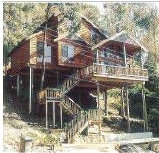
Figure 67 Example of a pole house on sloping land (Source: Practical Pole Homes)
