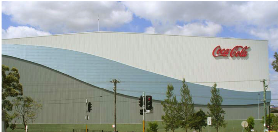
Picture 1: High Bay Warehouse Façade
