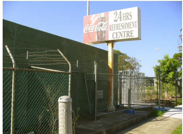
Picture 6: Refreshment Centre sign with overall height of 4.5m and illuminated panel 2.2m (w) x 1.2m (h)
