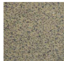
Exposed Aggregate Finish for landscape paved areas at drivers amenities and dry creek areas
