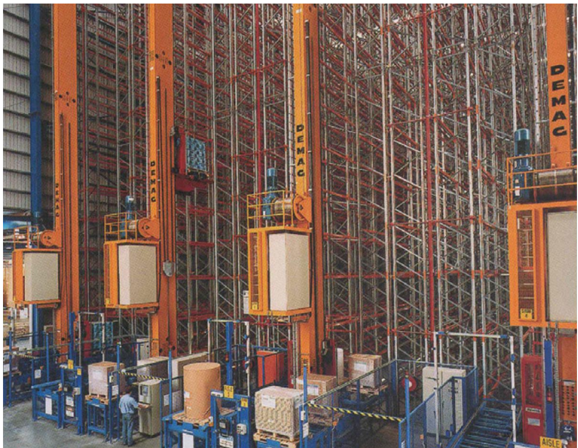
Figure 13 – Interior of a High-Bay Warehouse
