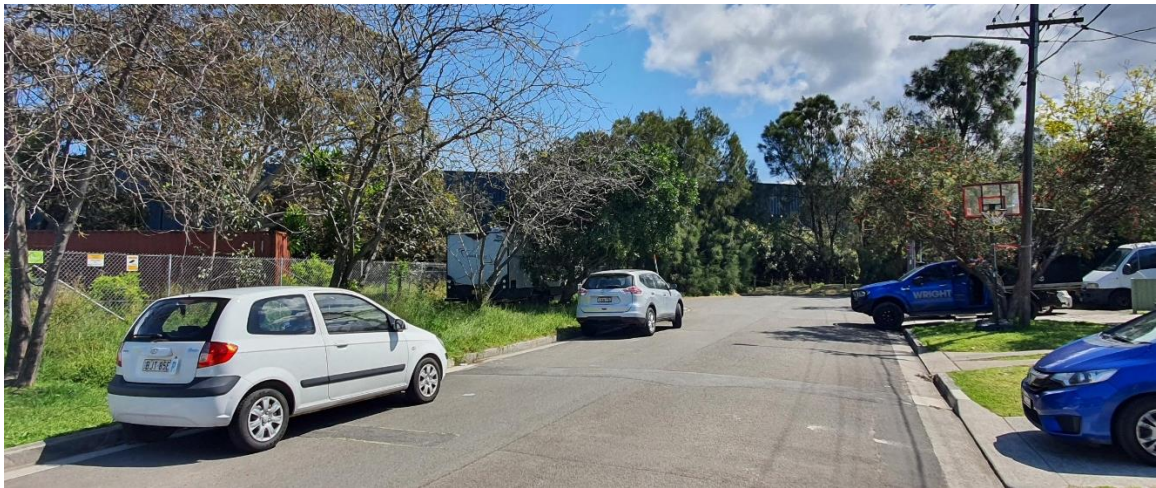
Figure 13. View of the existing noise barrier from western end of Partanna Avenue looking east. Photo taken by WSP, Oct 2022.
