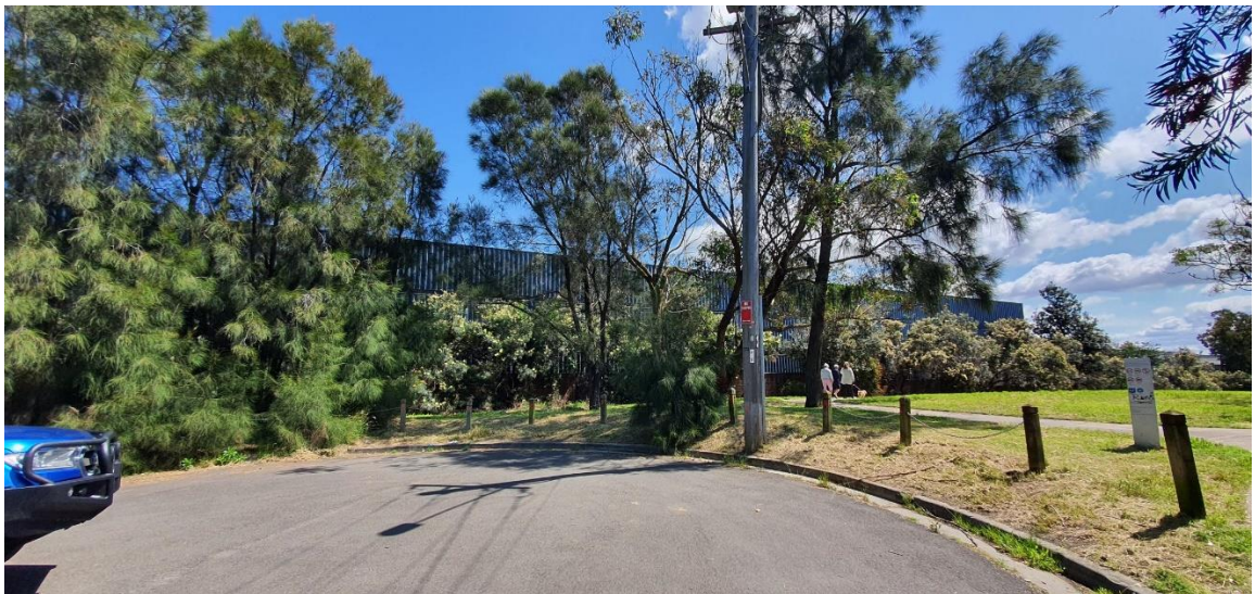
Figure 14. View of the existing noise barrier from western end of Partanna Avenue looking north-east. Photo taken by WSP, Oct 2022.
