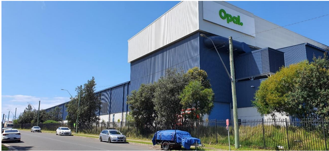
Figure 2. façade of the other site buildings on the corner of McCauley St and Botany Rd. Photo taken by WSP, Oct 2022
