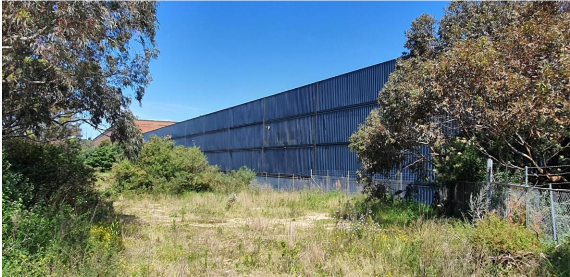
Figure 17. View of the existing noise barrier from the western end of Partanna Avenue. Photo taken by WSP, Oct 2022.
