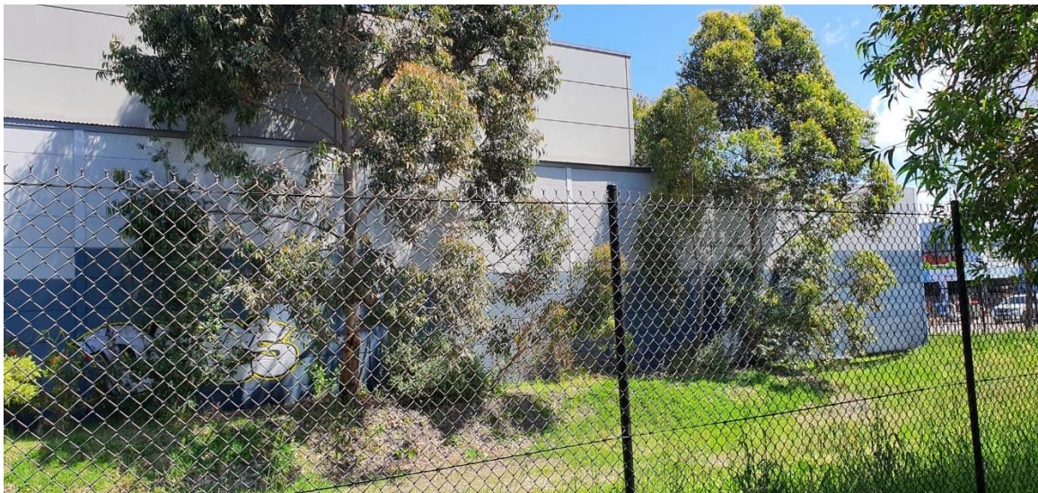
Figure 16. A closer view of the hebel block fence along the eastern boundary of the adjoining industrial site to the north, viewed from Purcell Park. Photo taken by WSP, Oct 2022.
