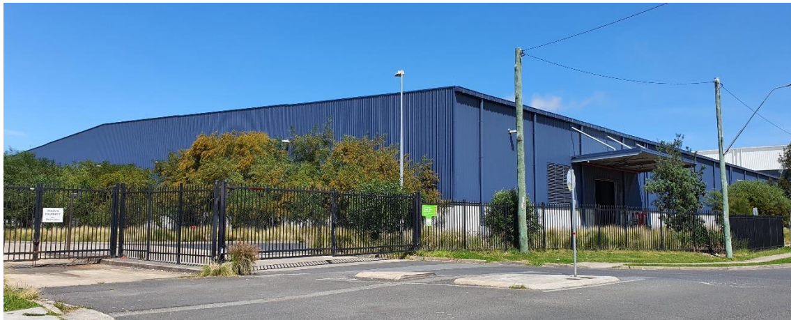
Figure 3. façade of the other site buildings along McCauley St frontage. Photo taken by WSP, Oct 2022
