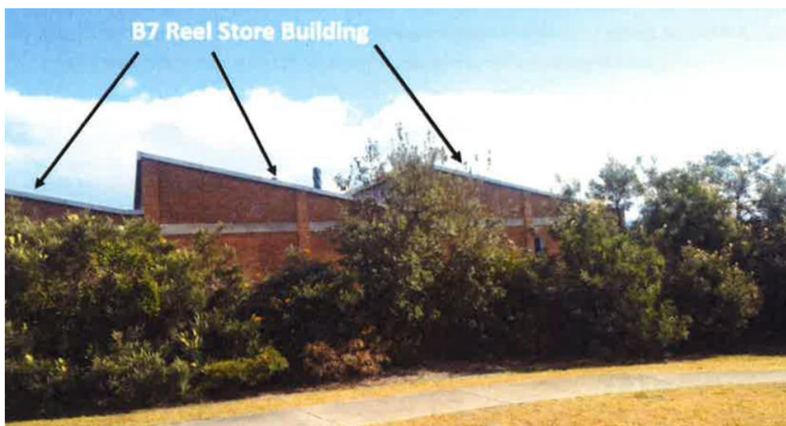
Figure 9. View of the pre-existing B7 reel store from the southern end of Purcell Park. Photo contained in the modification assessment report for MOD 8 application by DPE.
