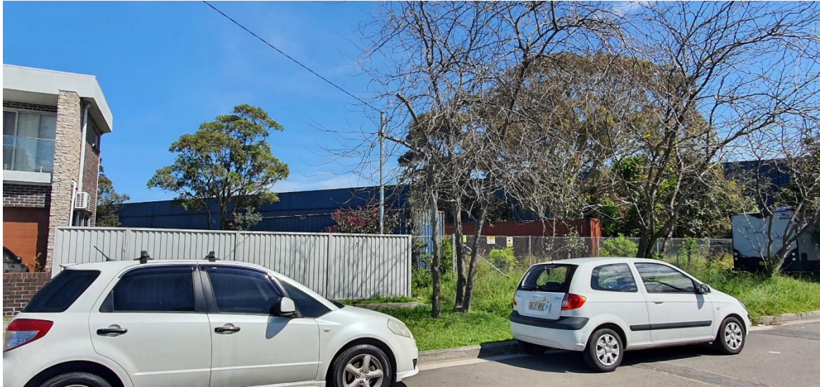
Figure 12. View of the existing noise barrier from western end of Partanna Avenue looking south. Photo taken by WSP, Oct 2022.
