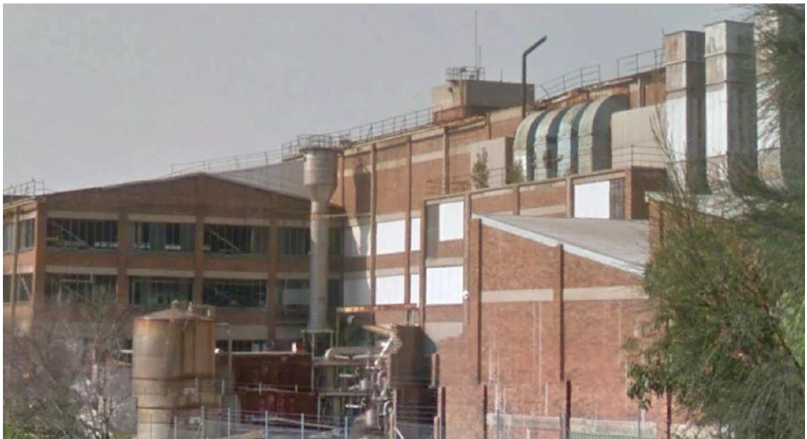
Figure 7. View of the pre-existing B7 paper mill and reel store on site, visible from Purcell Park. Photo contained in the noise management report by Hutchison Weller dated 19 Sep 2016.
