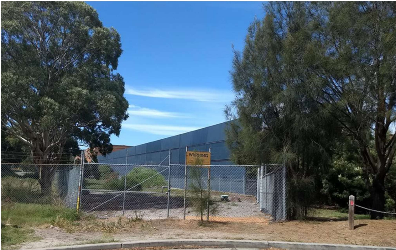
Figure 2 Paper mill (southern section) container noise wall - March 2018
