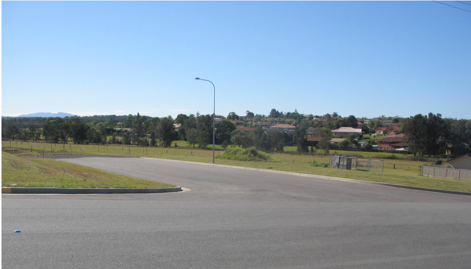
Figure 1 Intersection of Road 1 with Banyula Drive looking north - constructed 2005
