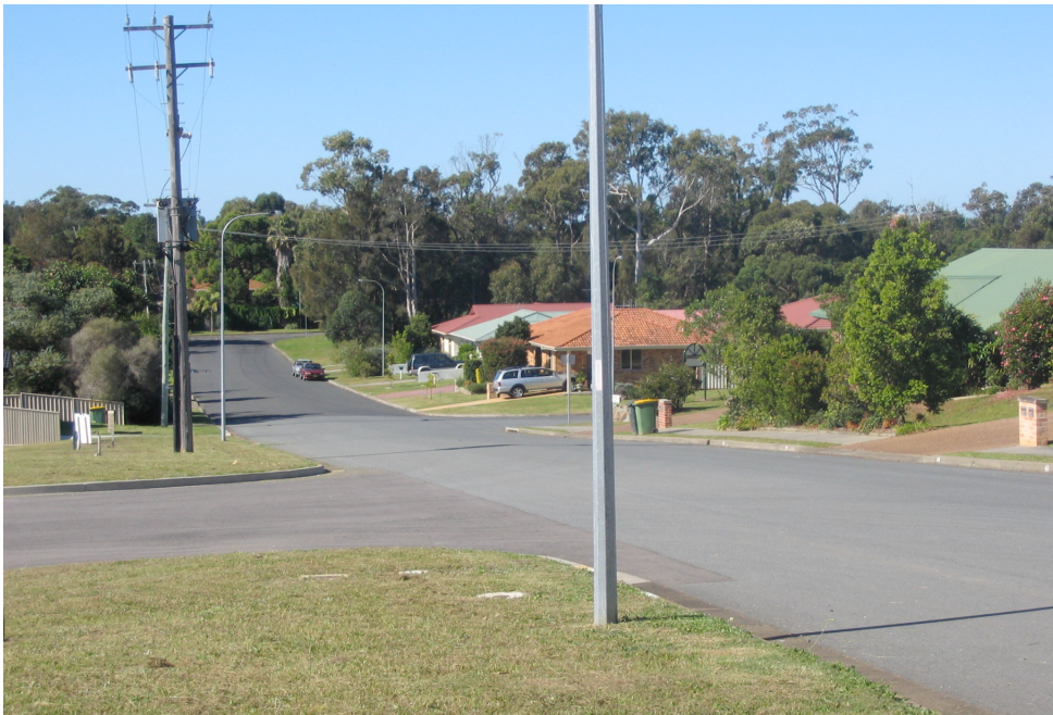
Figure 2 Intersection of Road 1 with Banyula Drive looking east - constructed 2005
