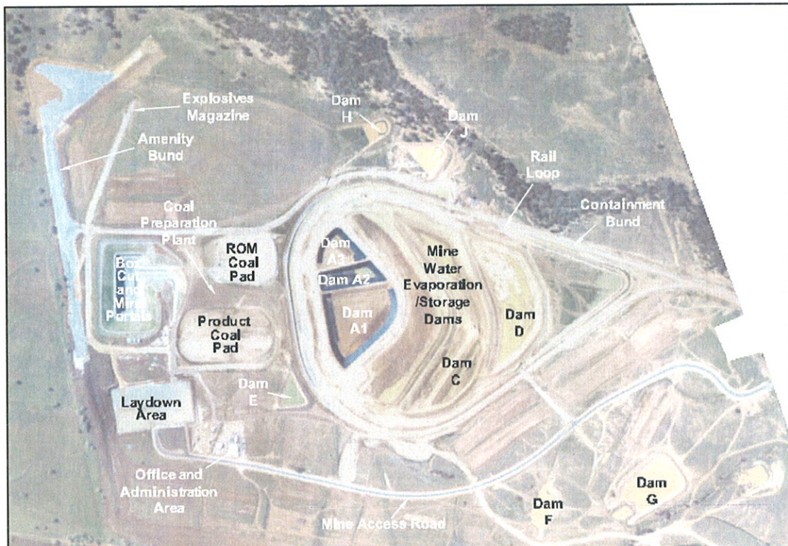
Figure 3: Aerial View of Stage 1 Pit Top
