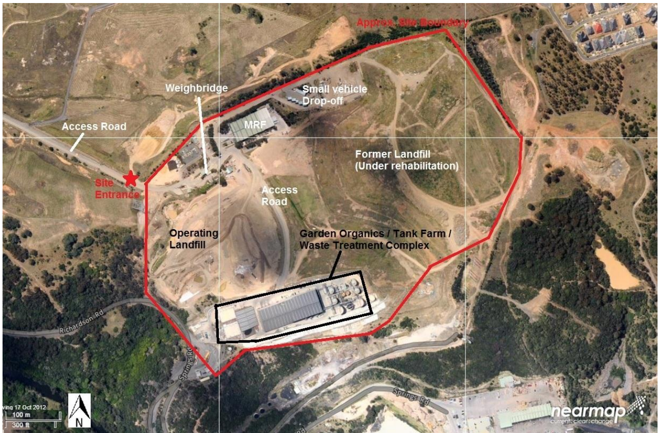
Figure 1.1 The Spring Farm Resource Recovery Park Site
