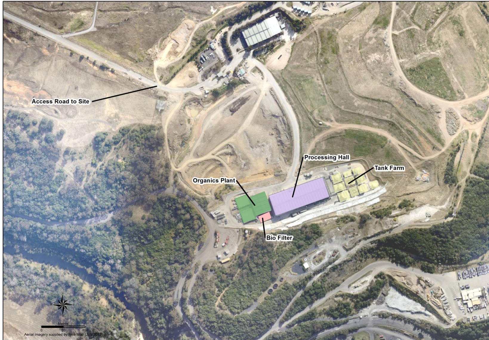
Figure 2-2 Existing infrastructure of the ARRT Facility
