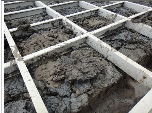
Top of UASB before cleaning
