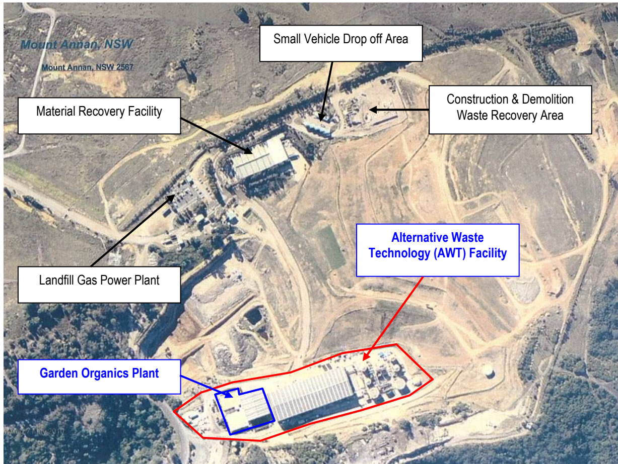
Figure 2: The Garden Organics Plant (GOP) within the AWT Facility at the Macarthur Resource Recovery Park
