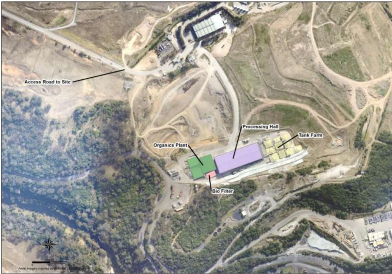
Figure 1 Existing Infrastructure of the ARRTF (EA, Cardno, 2013)
